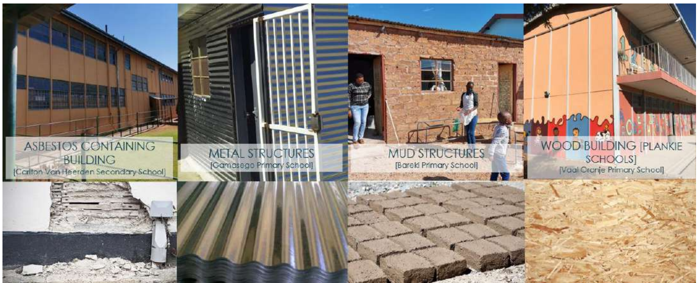
Figure 2: Inappropriate Structure Examples
